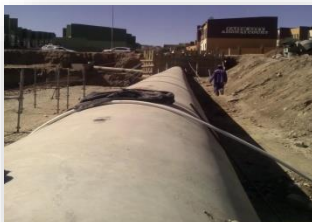
New Residential Development in Rocky Crest – 1050mmØ Storm water Pipe: Civil Engineering
